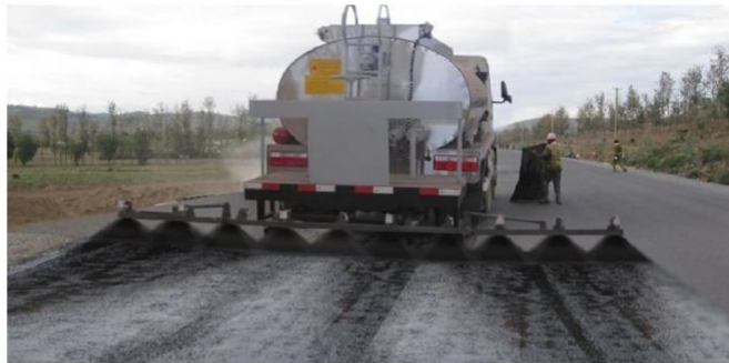
Asphalt truck working at site
